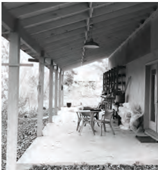
north shed view
