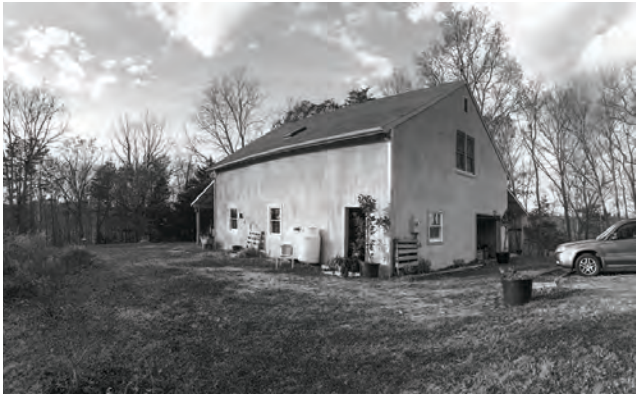
south west view
